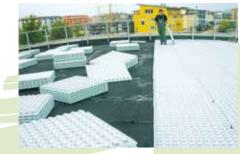
Once the Floratherm<sup>®</sup> elements were installed approx. 0,15 m of intensive substrate was blown onto the area.
