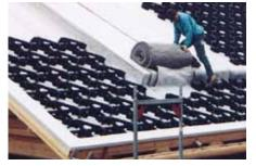
Once the area has been covered with the Protection Mat WSM 150, the Georaster<sup>®</sup> elements are installed, starting from the bottom up.
