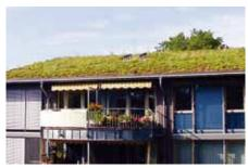
When dimensioning an eaves upstand or shear barrier, the decisive factor is not only the watersaturated weight of the green roof build up but also the estimated snow loads for the locality.
