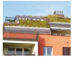
There is no standard solution for barrel roofs. However, solutions specific to your building can be worked out in conjunction with the ZinCo Technical Department, as seen with the roofs of apartment blocks in Pfäffikon in Switzerland (photo above). As gravel edge strips cannot be used for roofs with an extreme pitch, grass pavers ensure a solid and location-stable option for eaves drainage.
