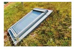
In the case of roof penetrations it is important to ensure that the waterproofing layer is drawn up to at least 100 mm above the upper edge of the substrate layer. Green roof build-ups can be bordered using the stainless steel Eaves Profile TRP 140 in combination with shear retainers (either Support Bracket TSH or Shear-Fix LF).
