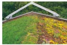
The type of vegetation that will survive on pitched roofs without additional irrigation can be seen in the three photos from the Gardening Department of the City of Tübingen, Germany (System Build-up "Pitched Green Roof" carried out in 1986). The turf rolls installed initially on the north-facing side failed entirely after a short space of time, while the Sedum-herb vegetation on the southfacing side (plant community "Rockery Type Plants") also took over the northfacing side.
