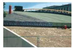
The transition area was covered with gravel and topsoil, in order to connect the roof with the natural ground underneath.
