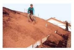
The system substrate "Heather with Lavender-light" is, e.g. delivered in a silo tanker. It is then blown onto the roof using a hose until the Georaster<sup>®</sup> elements are filled and covered up to about 10 mm over their upper edge.
