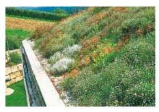
Even after only one vegetation period the plant coverage is largely complete. The roof area in this example is drained by means of an outer-lying gutter into which the three water spouts carry any excess water.
