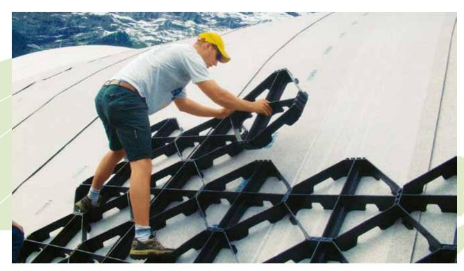
The System Build-up "Steep Pitched Green Roof" based on the ZinCo Georaster<sup>®</sup> system, as presented here, is suitable for greening roof areas with a pitch of over 25°. The Georaster<sup>®</sup> elements are 540 x 540 mm in size, 100 mm high and made of recycled polyethylene (HDPE). No tools are required to attach them to each other. The result is a stable and continuous unit.
