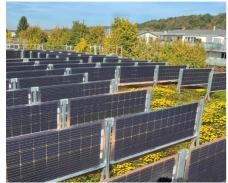
Base frame made of Magnelis specially designed for the vertical use of bifacial modules; matched to the ZinCo Solar Base® SB 200.
