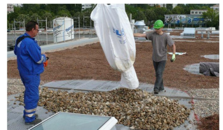
Visitor centre of the BUGA 2017: Creating a gravel area.
