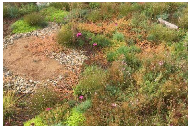
Roof of a hotel in Erlangen, Germany: temporary water/clay surface and species-rich greening.
