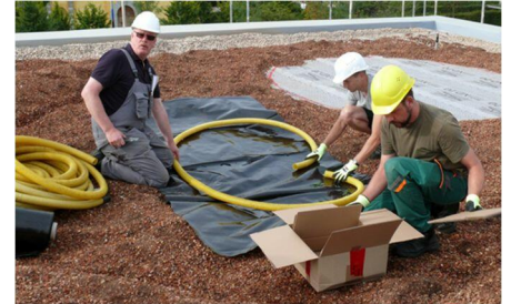
Visitor centre of the BUGA 2017: Here a drainage hose was installed as the edging of the temporary water area.
