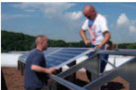
5. The solar panels are installed.
