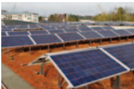
Mounting system east-west, type "Saddle".
