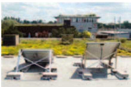
The difference in temperature of various roof build-ups was measured using a test installation on a ZinCo roof.
