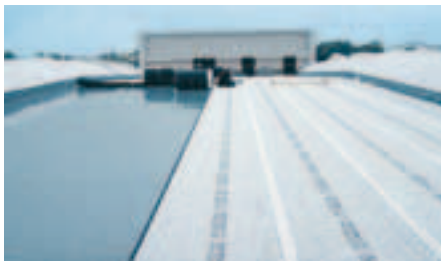
1. The roof membrane is covered with the protection, drainage and water retention element Fixodrain® XD 20 .
