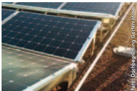
Mounting system east-west, type "Butterfly".
