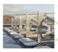
Either a solar energy system or a green roof? That was the past! With the system build-up SolarVert® (Fixodrain® XD 20, ZinCo Solar Base® and basic frame), the combination of solar panels and green roof achieve even greater efficiency. And, there is no need to penetrate the roof membrane as the load required to keep the system permanently stable is provided by the green roof itself. The solar bases can be placed wherever they are required on the Fixodrain® layer.
